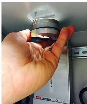
Figure 35: Secure retainer ring
